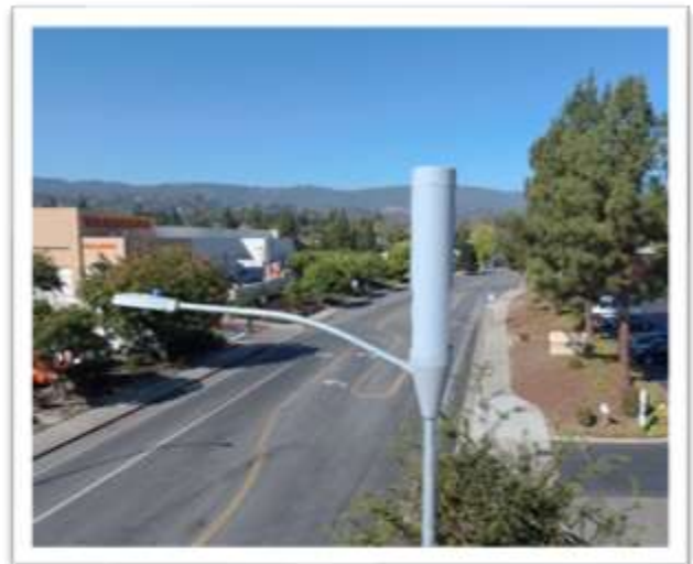
Figure 1 A Verizon gNodeB in Cupertino, California
